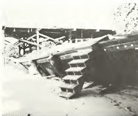
FIGURE 129.—Dislocation of an access stile surmounting the seawall at Malibu Beach, Calif., as the result of undermining and toppling of the wall by storm-amplified perigean spring tides on 1974 January 8.
